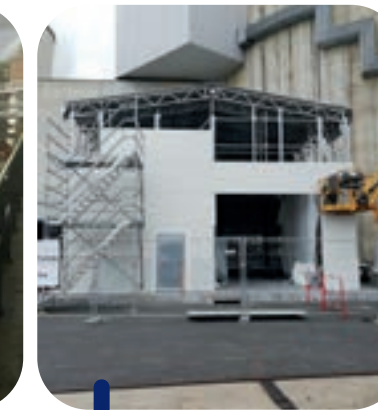
Cladded access structure CNPE Civaux
