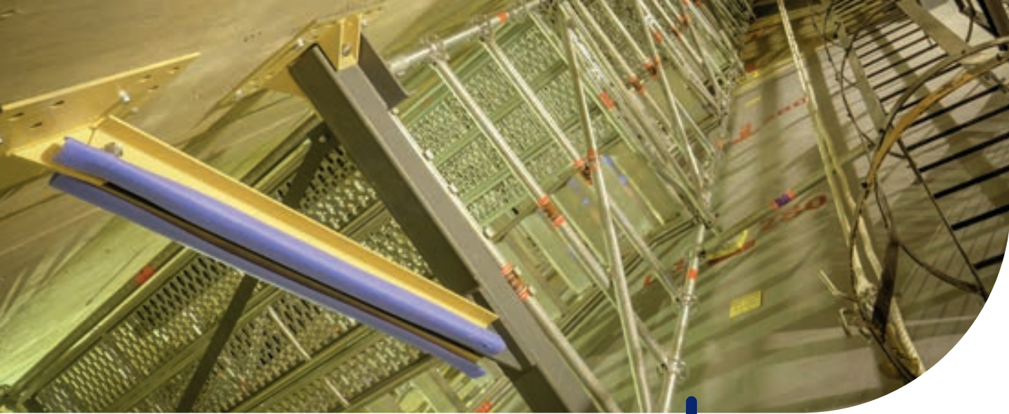
Means of access with design a specific support console Extrados CNPE Cattenom
