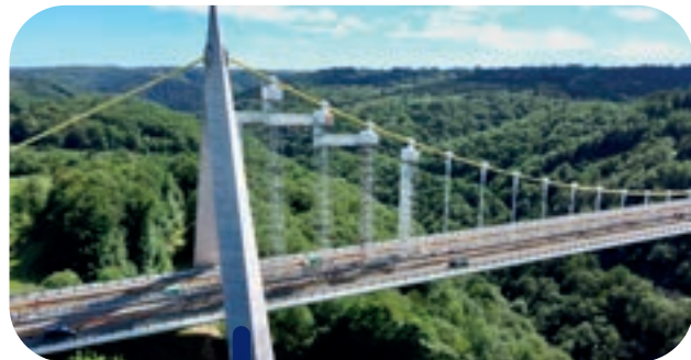
Access and containment Chavanon Viaduct
